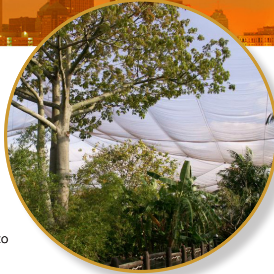
90,000 Square feet Stainless Steel Mesh.
